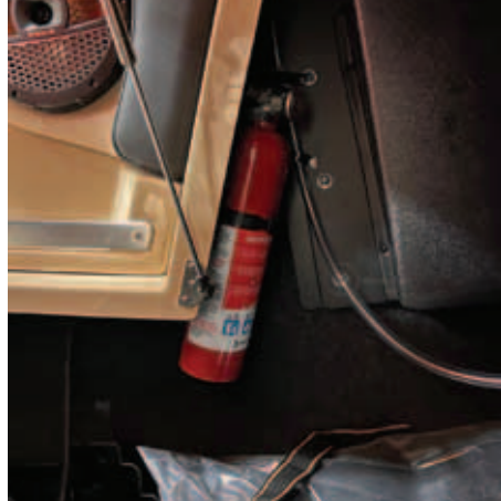
Handheld Fire Extinguisher
