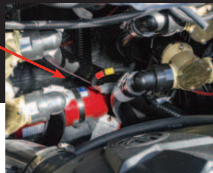
Location of Engine Fire Extinguisher
