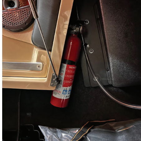
Handheld Fire Extinguisher
